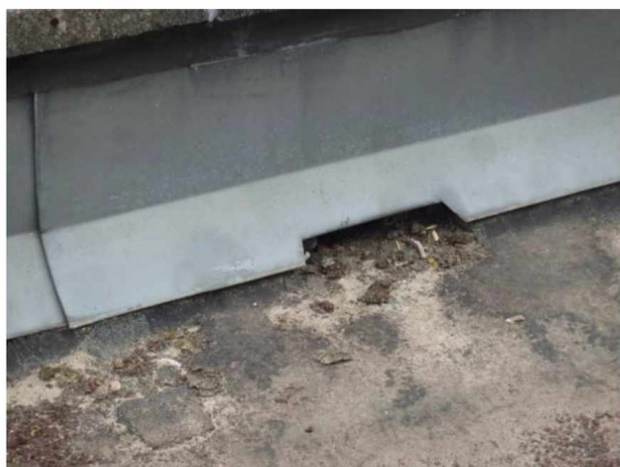
17: sparing in zinkwerk tpv hemelwaterafvoer
