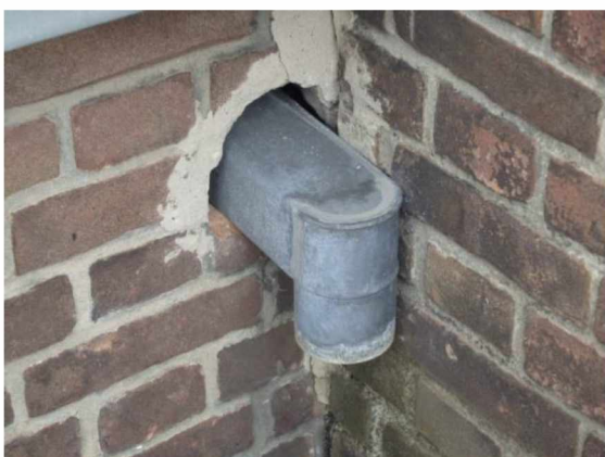
35: detail hemelwaterafvoer
